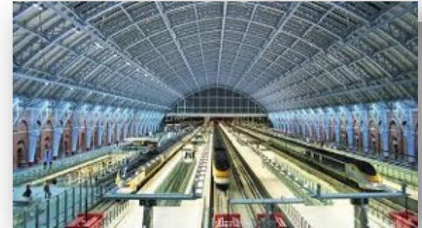
Roof panels of St Pancras Station in London (10000 m 2 , 18000 Glass panels) with TiO 2 ENM photocatalyst & Self-cleaning
