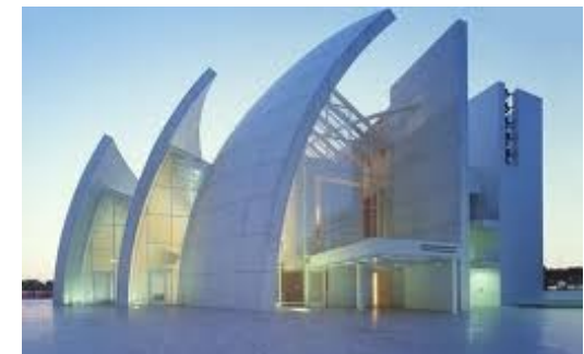
Church "Dives in Misericordia", Rome, made by using self-cleaning concrete
